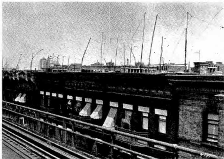
Even today antenna arrays similar to this can be seen in every large city.
